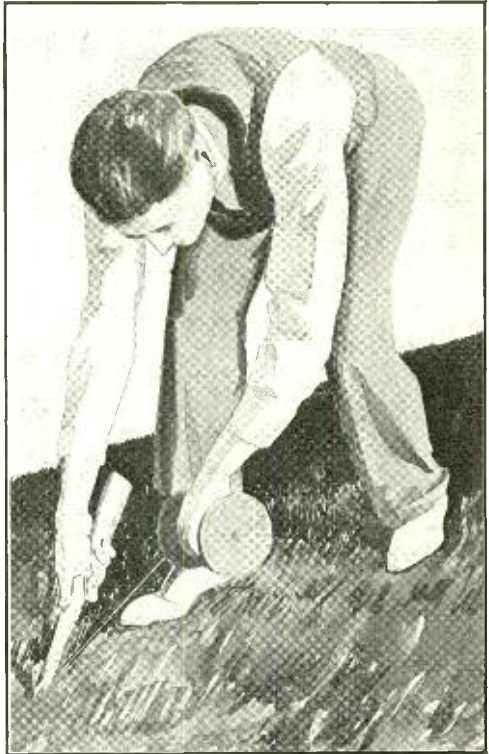
A buried ground wire is the basis of a new noise-reducing system. To lay the wire the author had wire spool in one hand and guided the wire in grooved plywood to force the wire into the ground. The method supplanted axe for handplow (above).
